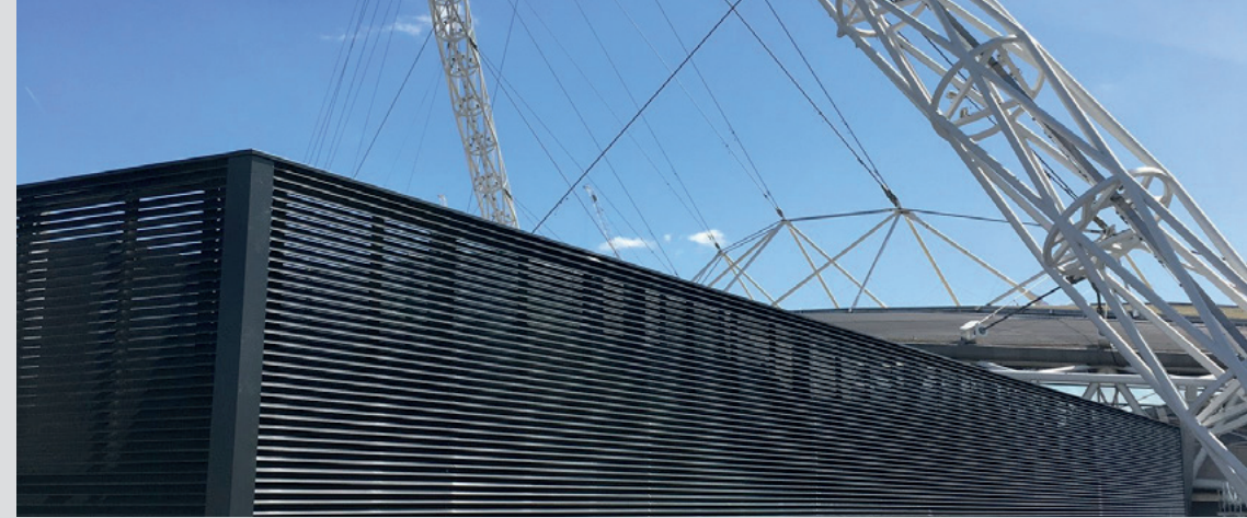
Wembley Stadium, London. Product 1UL/SH screening louvre.
