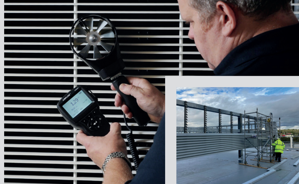
Above: Checking airflow on installed louvre panel. Right: Installation of 1UL/DH louvre.
