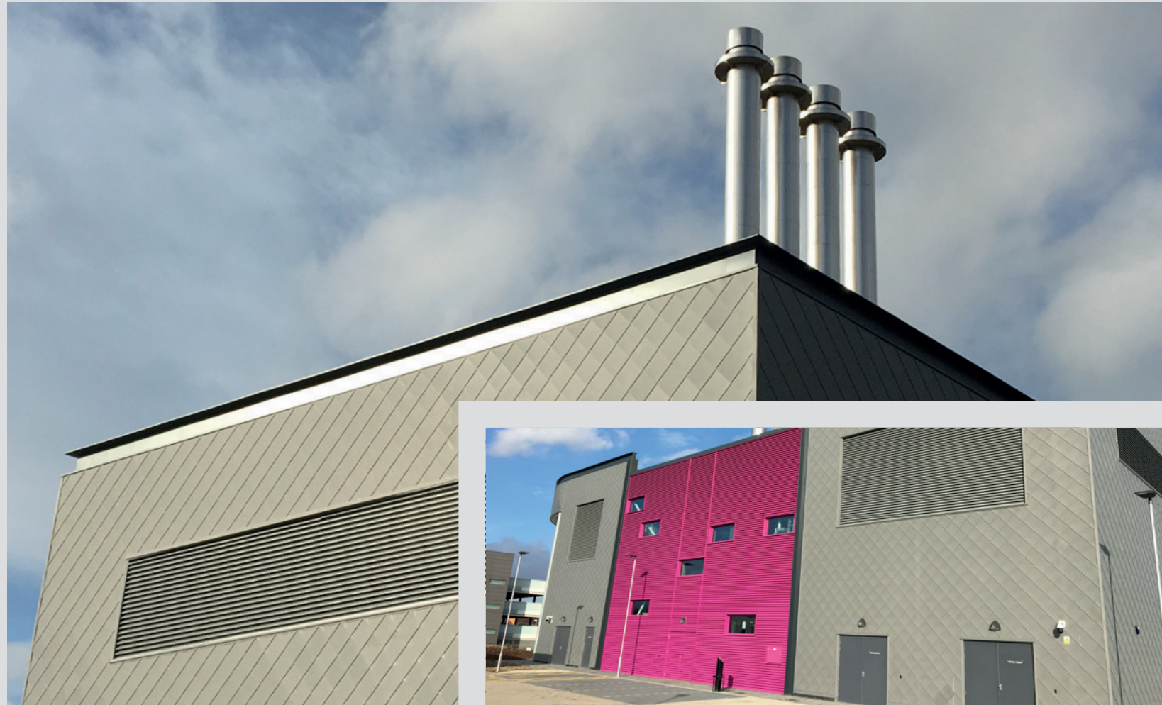
Right: Gateshead Energy Centre, Tyne & Wear. Product 2UL/DH.
