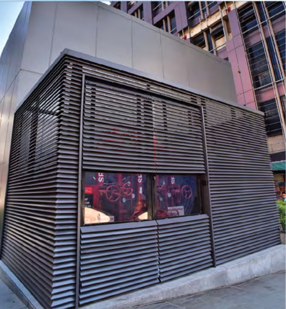
Project MRT Line 1 - Bukit Bintang & Intervention Shaft 2
