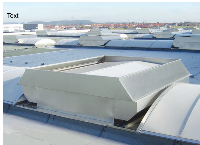
Apollo (see upper image) provides both smoke ventilation and environmental / day-to-day ventilation.
